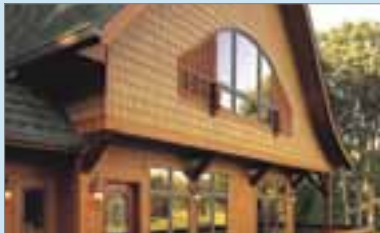
Fiber Cement Siding
